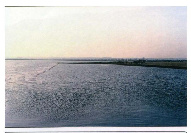
Plate 9. Bank-full situation showing waves breaking on front wall and wave refraction through the spillway
