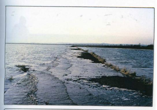
Plate 5. The surface of the set-back area is covered before waves break over the front wall
