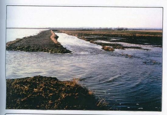
Plate 6. Early rising tide showing current flow around the edges of the spillway and into the front borrow pit
