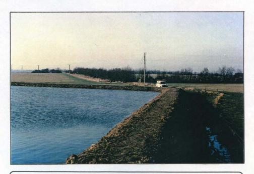
Plate 12. High tide at the east end of the site showing seepage through the eastern wall
