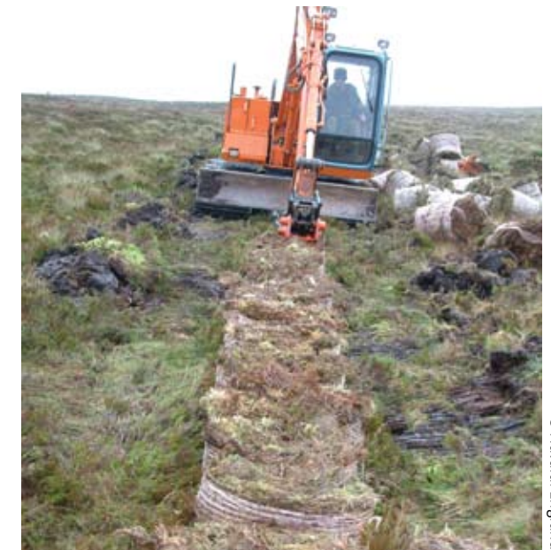
Blocking grips to restore upland peat – an important carbon store
