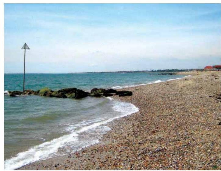
Replenished shingle material and rock groynes at Lee-on-the-Solent. Fine sediments imported with the shingle were selectively transported offshore and deposited as a thick drape over the interest features. Dave Evans/English Nature
