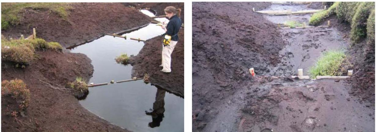
Figure 3-36: Infilling a gully with vegetation after the installation of plastic sheet piling (from Evans et al., 2005)
