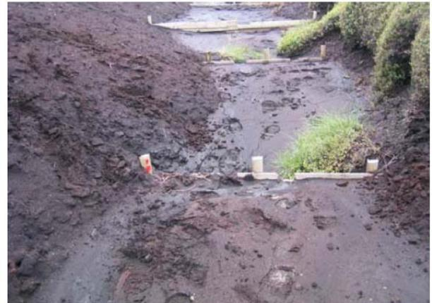
Figure 3-36: Infilling a gully with vegetation after the installation of plastic sheet piling (from Evans et al., 2005)
