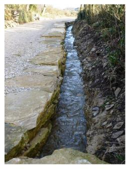
Over time the Priest's Way suffered from our changing weather/climatic conditions, increases in rainfall and varied land use and land management. This resulted in water run-off from adjacent fields that caused erosion in certain locations and seasonal flooding. At its worse it was difficult to travel along or totally unusable during the "rainy season" due to large expanses of water, deep gullies and mud. This made the route very unpleasant to use and often prevented people from using it.
