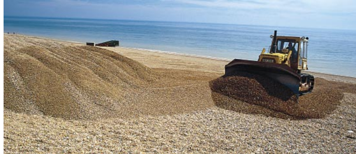
Re-profiling shingle with a bulldozer. Peter Wakely/English Nature
