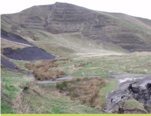
Mam Tor near Castleton and its famous landslide. Repeated slips caused the final closure of the road in 1979.
