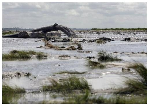
Figure C.2. Sediment being pumped into a realignment site.
