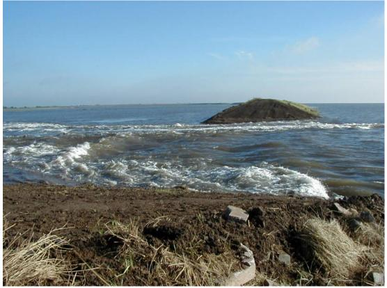
Figure C.7. Breach at flood tide.
