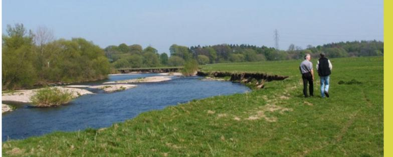
River Swale at Great Langton: The floodbank has been set back from the river here, creating temporary flood storage, wet grassland and natural features such as shingle banks, and allowing the river to meander in its floodplain.
