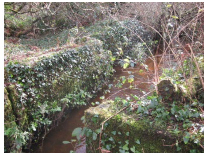
Photo 4: SP2, showing concrete channel and historical sluice gate
