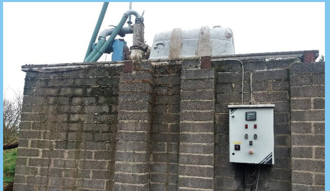
Slurry separator mounted on farm-constructed housing to save costs / provide covered storage area for separated solids.
