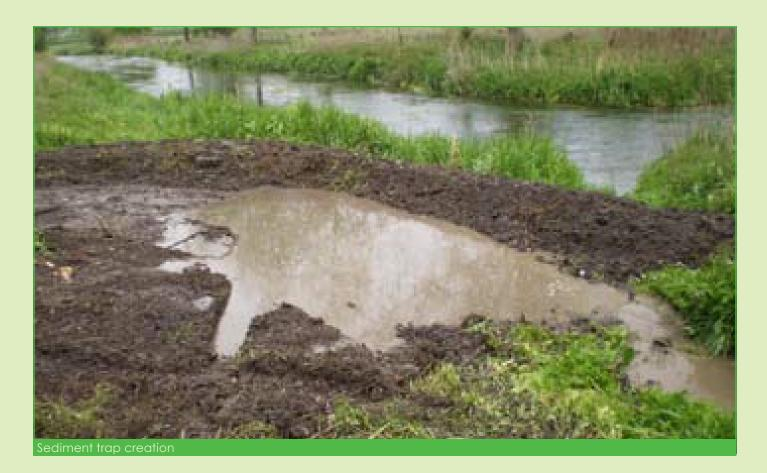
between the sediment trap and the river bank vegetation. Due to the connectivity provided by the highway, the sediment trap was not designed to hold all runoff, but to capture the first flush. Once vegetation establishes in the base and newly formed bund, this will provide additional filtration.
