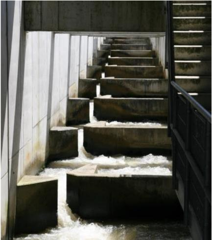
Figure 2.4. An example of a large vertical slot fish pass on the River Rhine that facilitates the passage of allis shad upstream of the 10 metre high lffezheim Dam.
