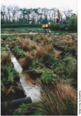
Figure 20: Pipe inlet from the neighbouring river to provide a constant water supply
