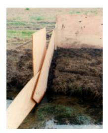
Figure 14: Plywood dug into the banks to cut off intersconnecting burrows prior to trapping.
