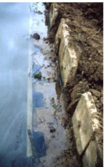
Figure 8: Concrete piling with gaps to provide 'bays' of damp earth, steel piling to water level
