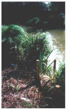
Figure 7: Coir rolls pinned with willow poles, with no other bank revetment
